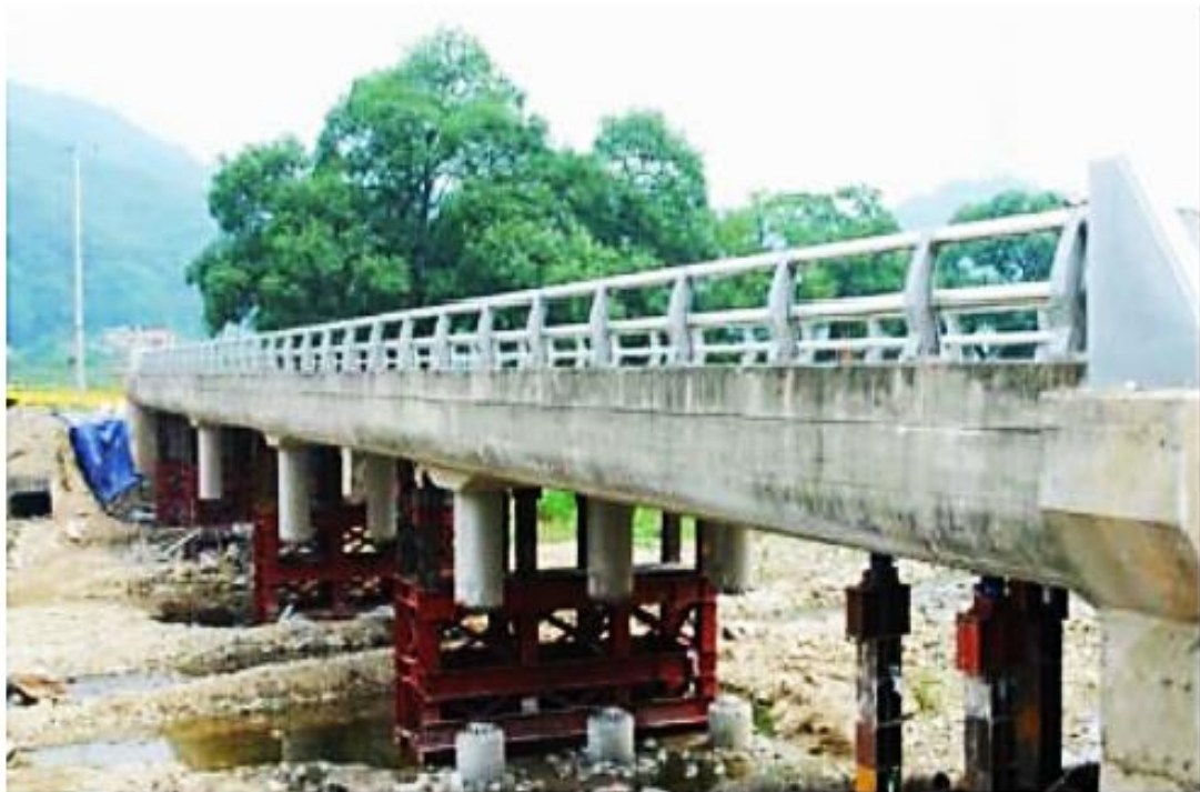
Figure 5: Retrofit of In-Service Bridges Source: Korea Expressway Corporation
